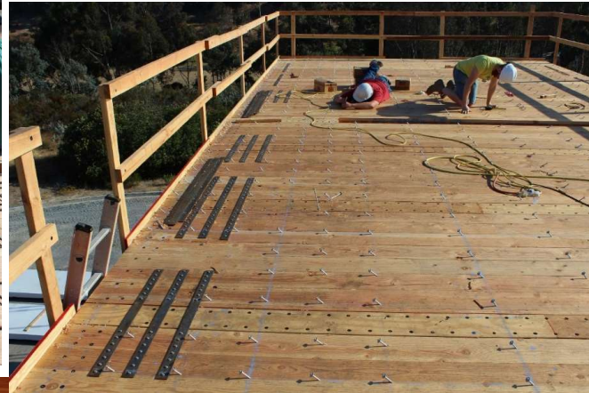
Rocking wall base detail
